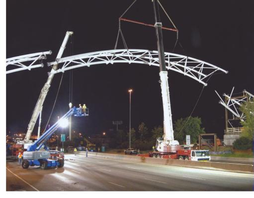
were suspended with temporary cables prior to installation of the permanent 1.5-in.- to 1.75- in.diameter cables. Because of the asymmetric layout and varying lengths and angles of the permanent cables, the deck girder geometry was set with a cambered twist, so that once the deck was poured it would match the proper geometry. The cable forces
