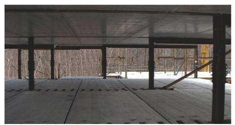
Unobstructed ceilings with Girder-Slab system.
