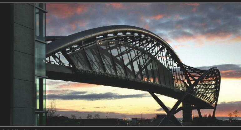
Helix Bridge, Seattle Washington. 36" O.D. x 1.25" wall and 24" O.D. x 1" wall bent to a multiple radius helix.
