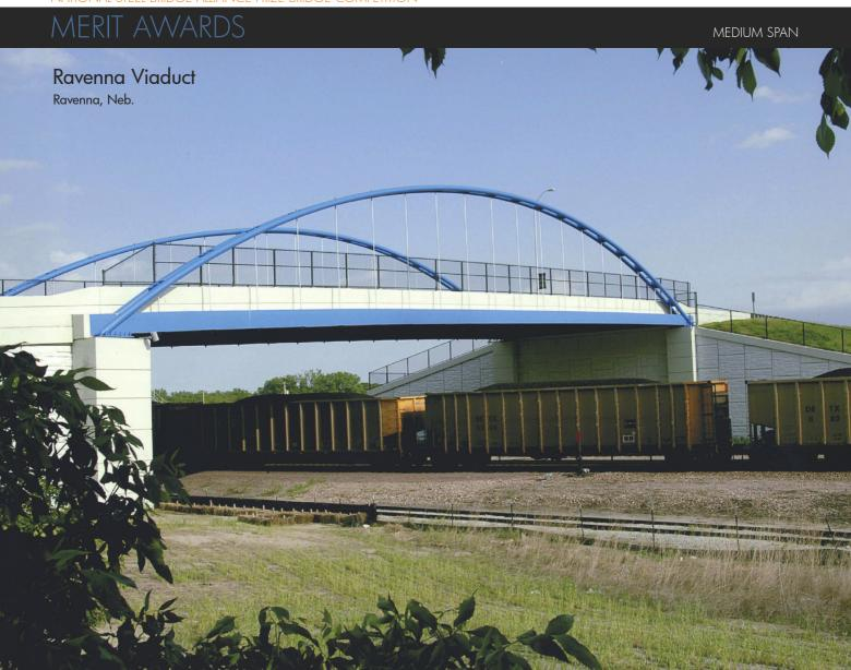
avenna viaduct is located on Highway 68 at the southern edge of downtown Ravenna, Neb. and spans a major route of the Burlington Northern Santa Fe Railroad. The original viaduct, built in 1937, was a five-span 265.5-ft.-long bridge with a 24-ft.-wide roadway and a 5-ft.-wide sidewalk. Thanks to structural deficiency and functional obsolescence, it was replaced with a new 174-ft. single-span parallel tied arch viaduct with a 43-ft.wide roadway and 8-ft.-wide sidewalk.
