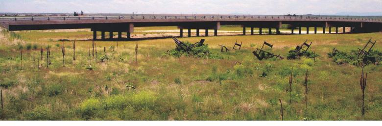
ust a few miles east of Denver, an innovative six-span bridge crosses Box Elder Creek on U.S. Highway 36 in Watkins, Colo. The new bridge, which replaces a previous one, is 470 ft long and 44 ft wide, and carries two lanes of traffic. The project's total cost of \$2.1 million includes removal of the old bridge, construction detour, and landscaping.
