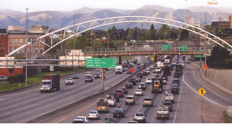
he new Highland Bridge restores a vital link between downtown Denver and the revitalized Highland neighborhood to the northwest. It replaces the 16th Street viaduct, a reinforced concrete viaduct that was failing when it was demolished in 1993, with a user-friendly pedway. It is the third in a family of three signature pedestrian bridges extending the city's downtown 16th Street Pedestrian Mall alignment across the Central Platte Valley.
